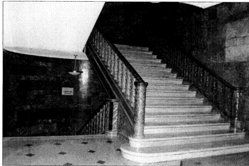
The Old Dearborn Bank Building lobby showing curving marble walls, terrazzo floors, marble stairs and highly ornamented metal railing. This grand staircase leads up to what was once the 2nd floor banking hall and down to the building's basement, which originally contained the vault and board room.
